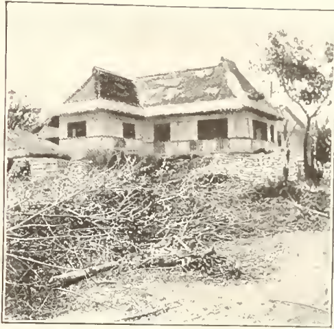
A HOUSE USED AS A BLOCKHOUSE, NEAR MANILA
